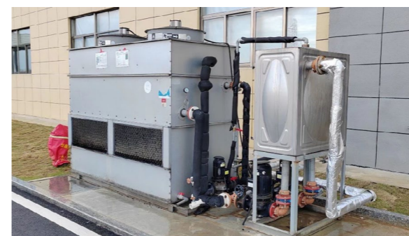
▶ New closed cooling tower
